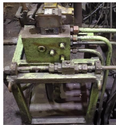
The valve after cleaning.
